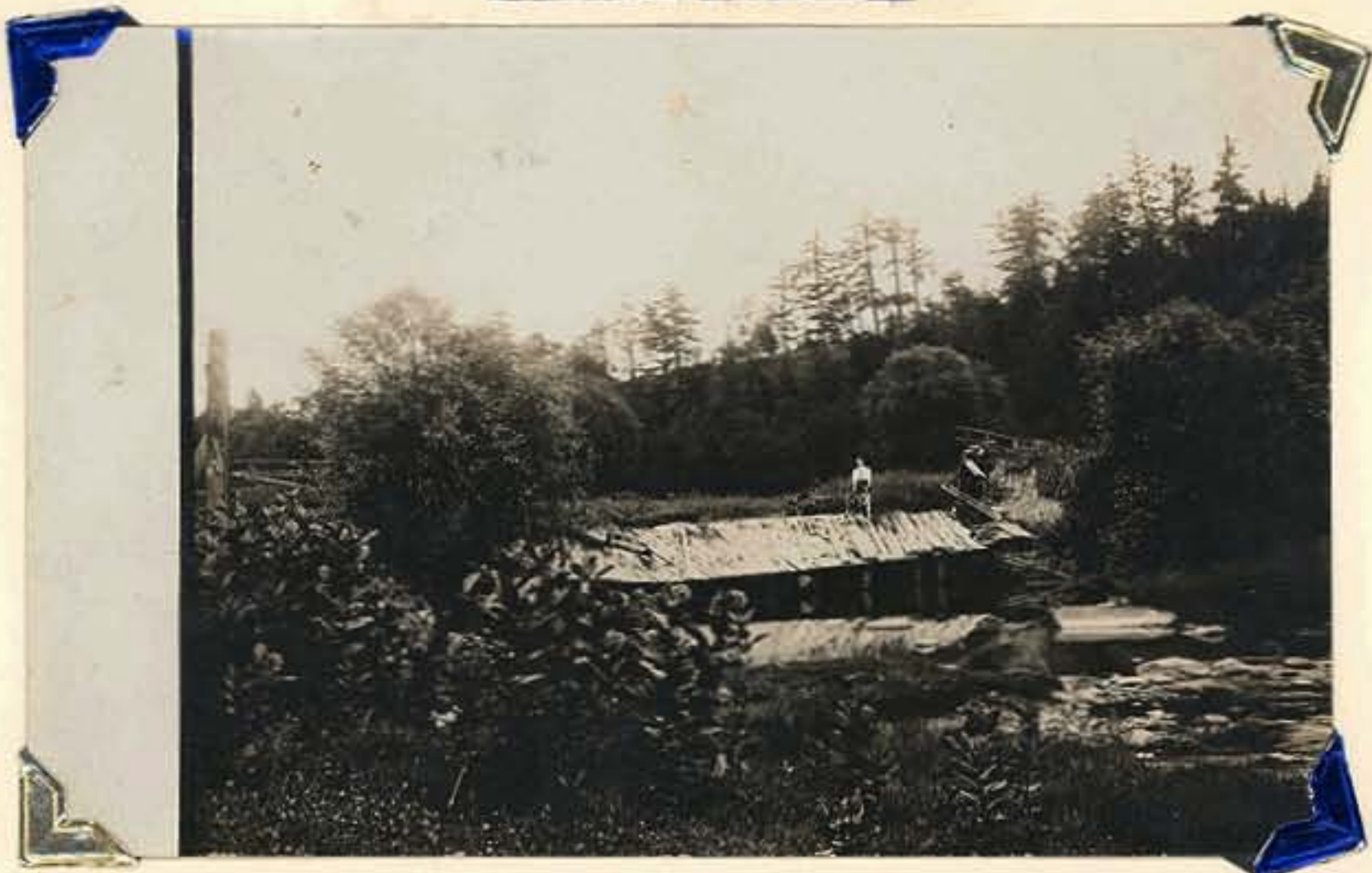
Picture of dam taken from bridge facing toward the East. Taken approx. 1910 - Mary Teasdale is standing on dam.
