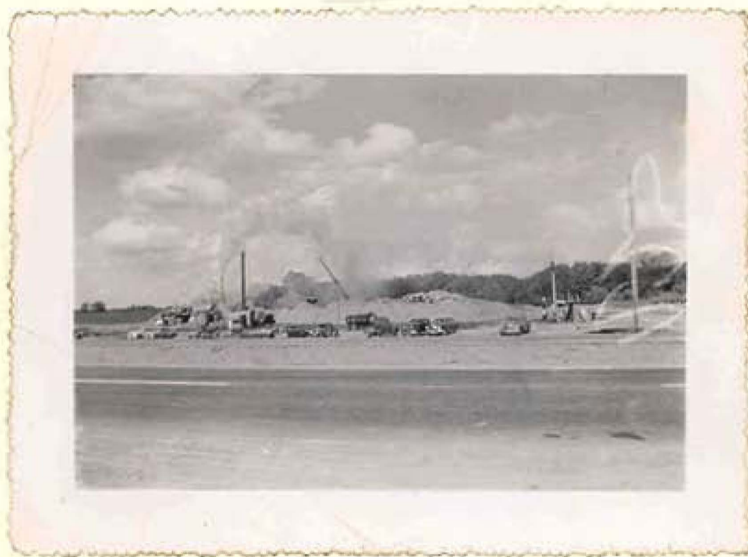
Beginning of service station - 400 Highway & King City Sideroad.
