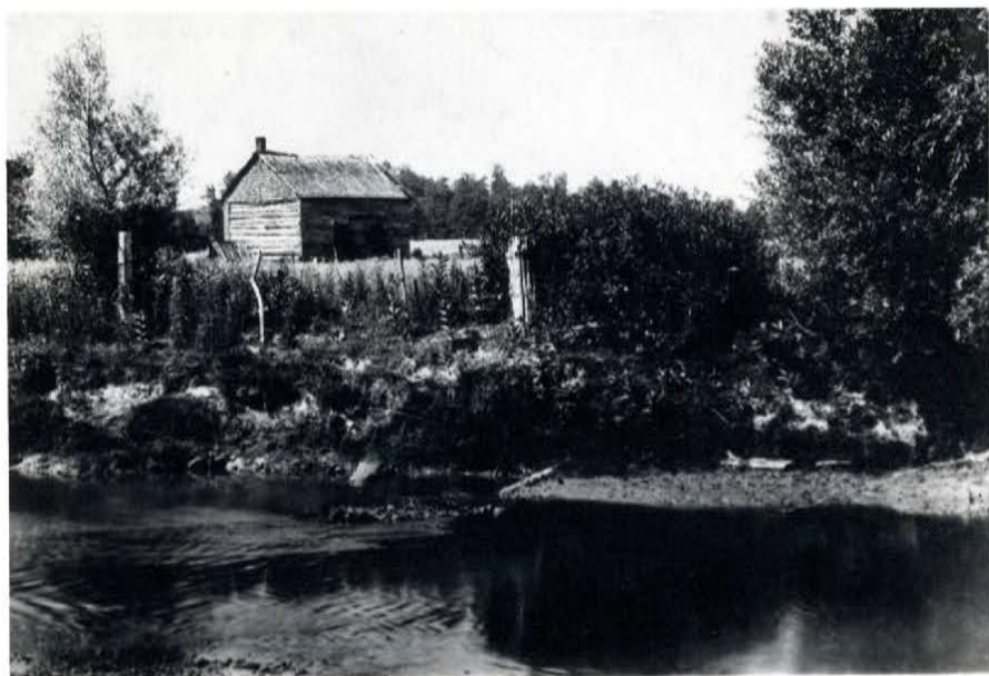
The log house built in 1881 on Lot 2 Con. 11 King Township by Wm. Jewitt
