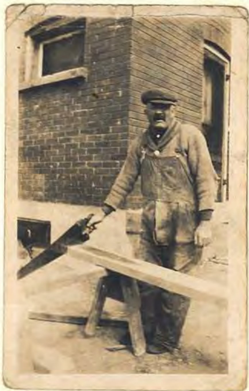
Ben Beynon building his house.
